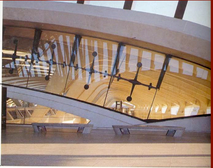
Concrete portal arches and platform access
