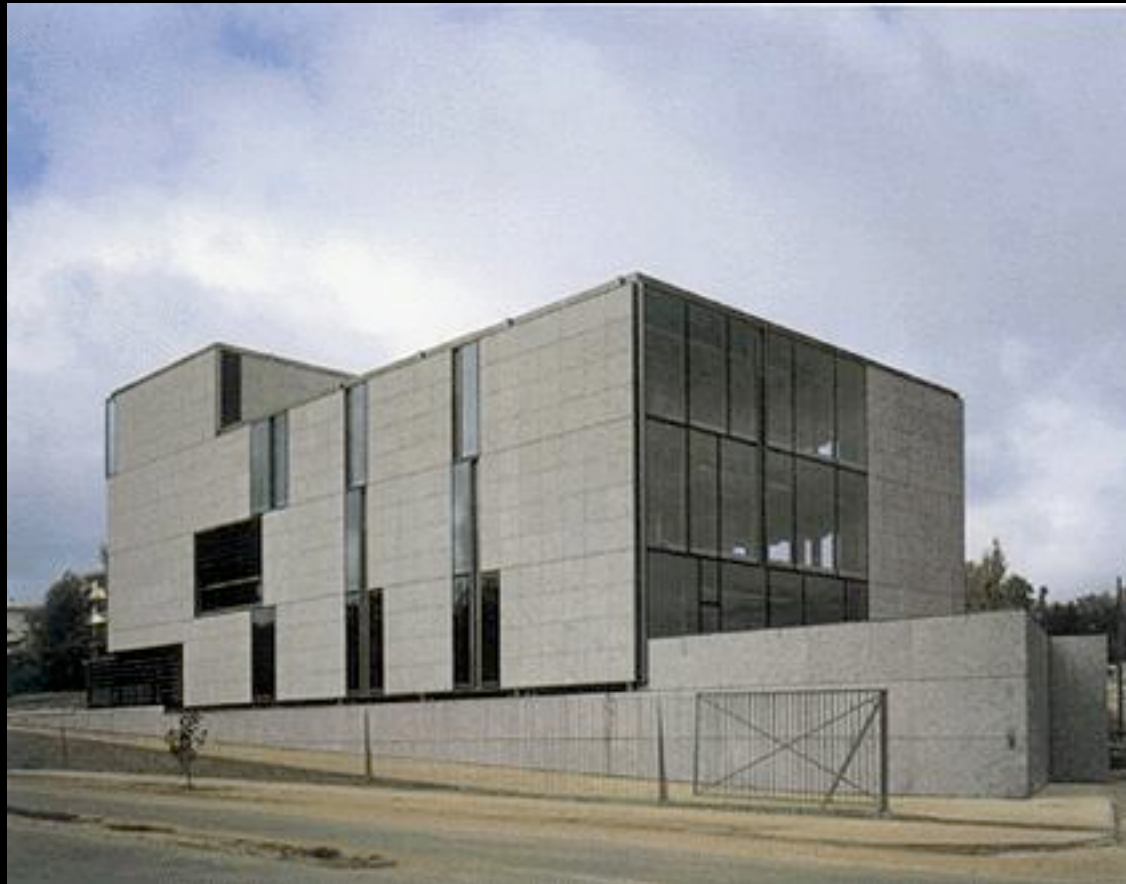
INEM Office Building Caceres, Spain
