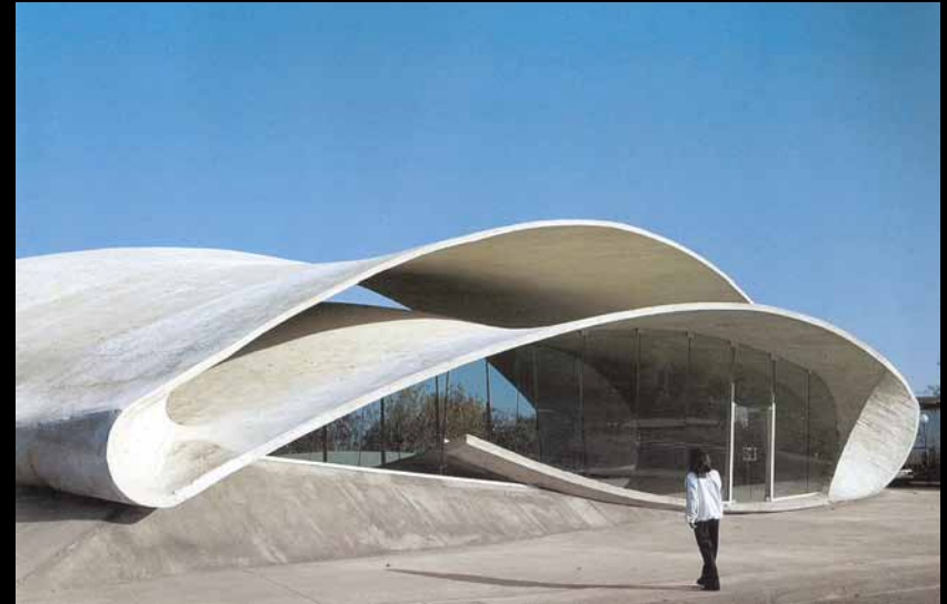
Subregional Bus Station
