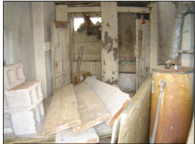
Interior Holt Addition Showing Restrooms
