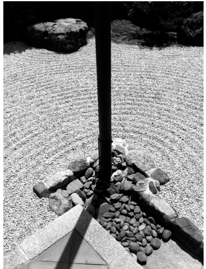
Zuiho-in (Daitokuji) / downspout detail Photo: Tsubaki ©
