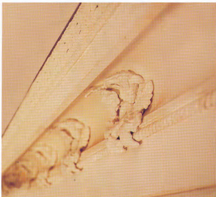
FIG. 36 PLASTER MOLDINGS, ROBINSON SINCLAIR HOUSE, GARDEN DISTRICT
