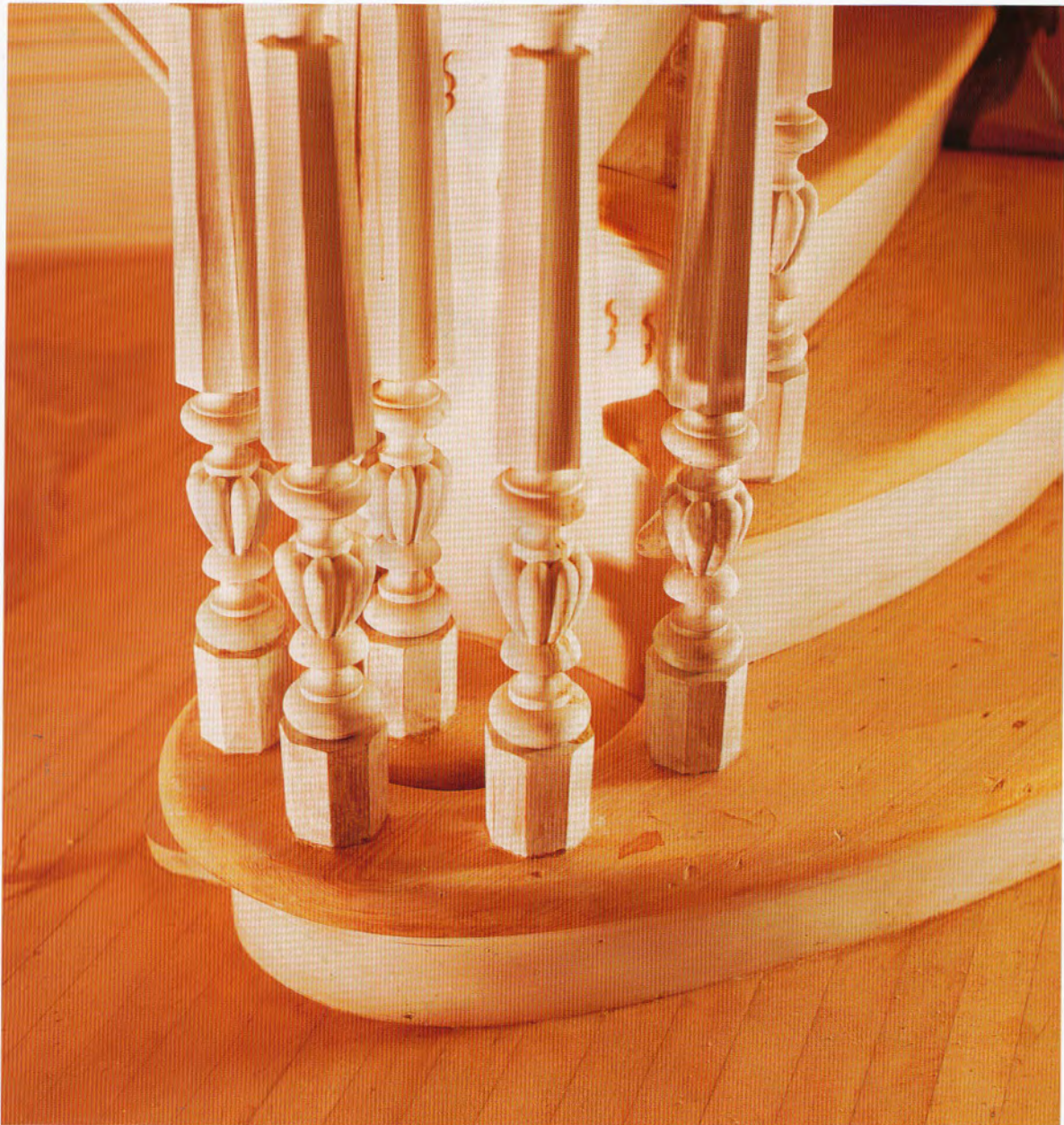
FIG. 24 STAIRWAY DETAIL, ROBINSON SINCLAIR HOUSE, GARDEN DISTRICT
