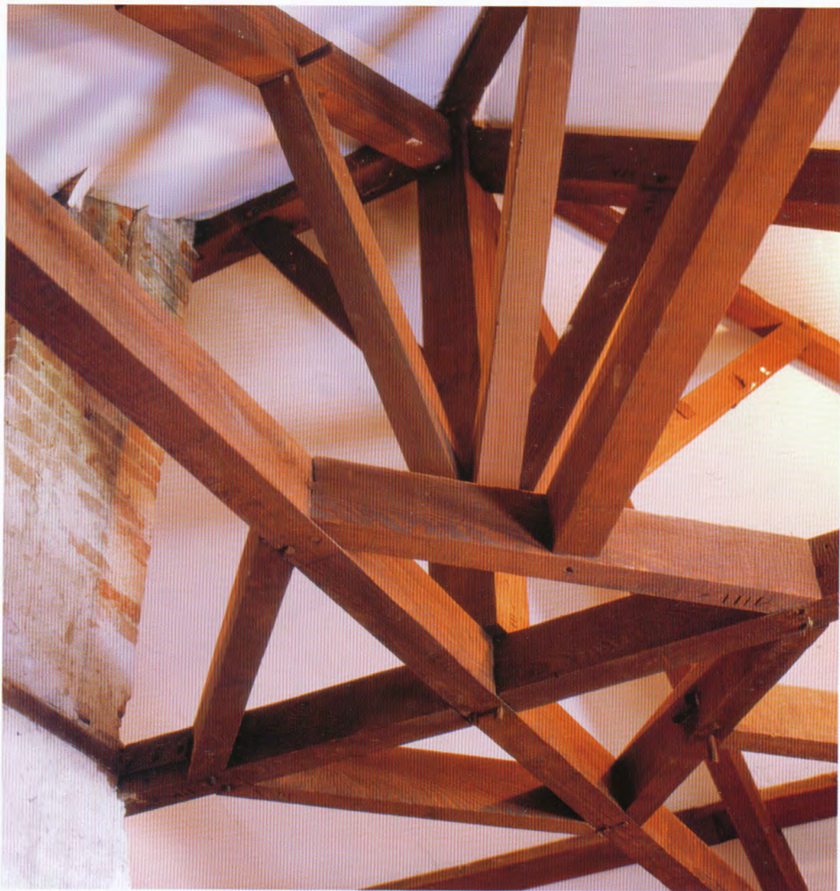
FIG. 16 MORTISE AND TENON TIMBER FRAMING, LOMBARD HOUSE ROOF, BYWATER
