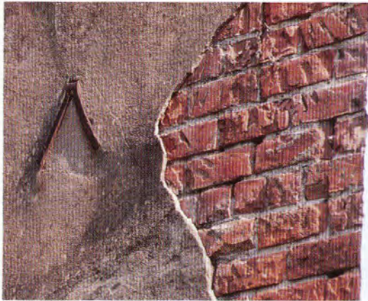
FIG. 27 SEALED SOFT RED BRICKS, MADAME JOHN'S LEGACY, FRENCH QUARTER
