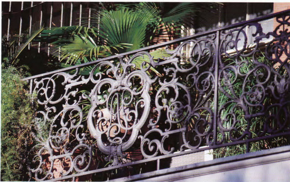
FIG. 38 PONTALBA BALCONY RAILING, FRENCH QUARTER
