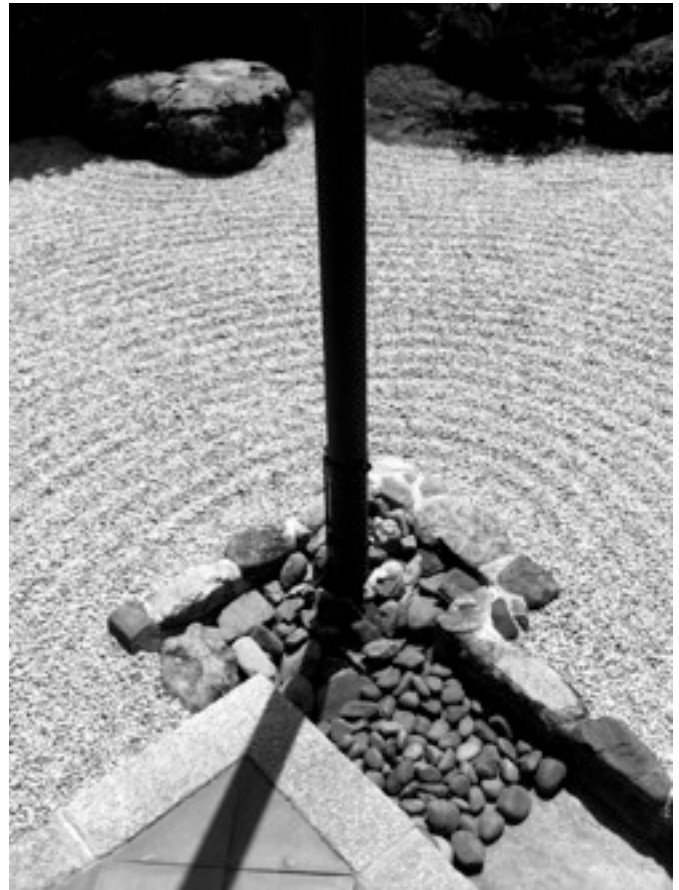
Zuiho-in (Daitokuji) / downspout detail Photo: Tsubaki ©
