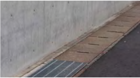
Slit and grate drainage in Naoshima
