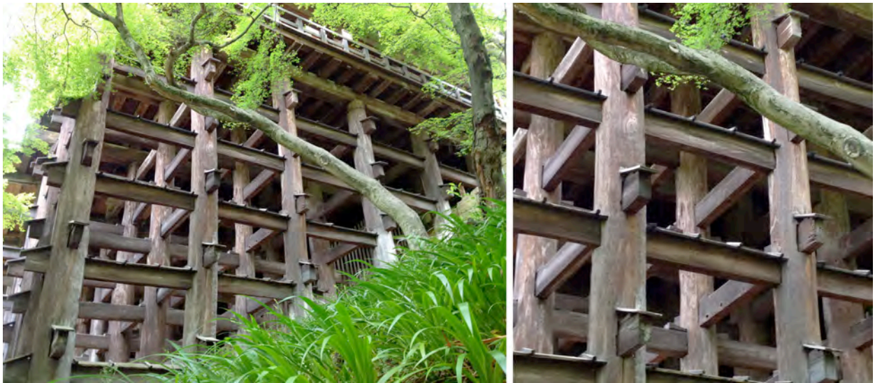
Support structure under Kiyomizu-dera temple, Kyoto, Japan.
